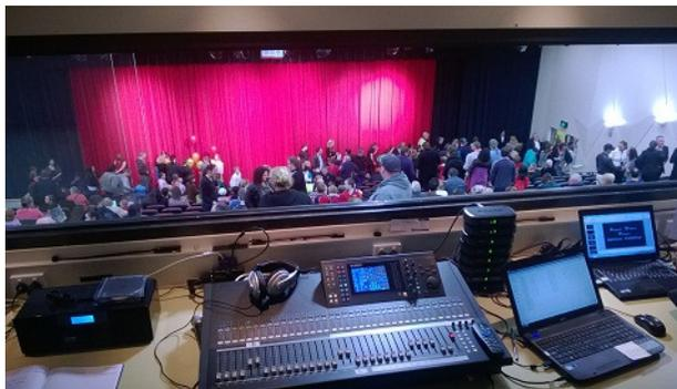
When the PAC was built the decision was made to provide for the future so a digital Yamaha LS9 32 channel sound desk was chosen. The entire building was professionally 'wired for sound' with stage boxes and patch bays throughout the building. We have a full compliment of vocal, instrument and wireless microphones to cater for almost any performance.
